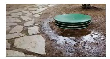
All septic tank soakaways have a limited lifespan which is made even shorter by the amount of suspended solids (little bits waste) in the effluent and they are eventually pushed out of the tank into the soakaway.
